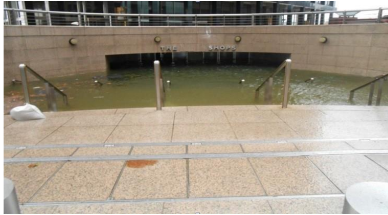
Hurricane Sandy brought the water level up over this shopping premises entrance.
